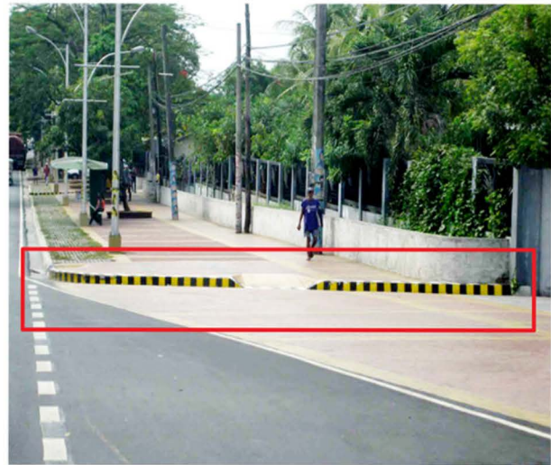
MARKINGS ON CURBS
