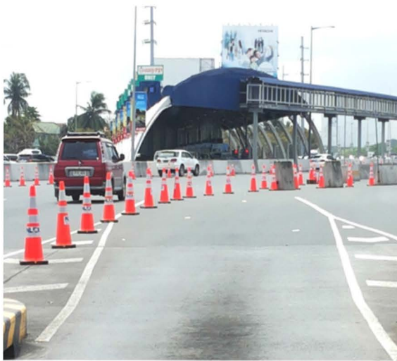
OBJECTS WITHIN THE ROADWAY
